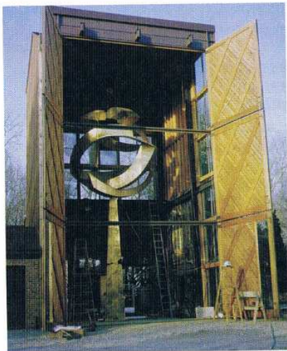
Welding can also be applied in the arts. Sculptor Jean Woodham created this 28-foot-high sculpture, which required a crane, cherry picker, and flatbed truck for installation.
