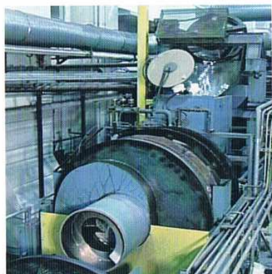
Blanks travel through a washing machine that removes impurities that are left after they have been heated.
